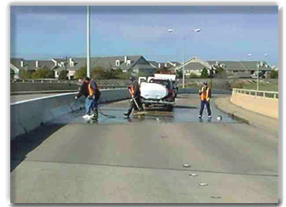
Collins Bridge - Richardson TX
