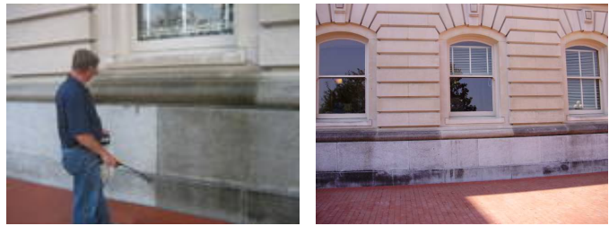
Application of Chem-Crete® Heritage CCC110 Treated area 3 years later
