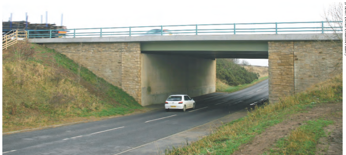
Figure 1: A motorway bridge situated on the A1(M) between junctions 60 and 61 which has been recently treated with Pavix CCC100.
